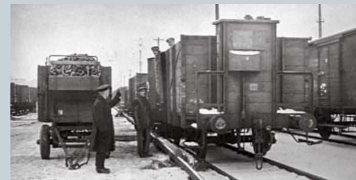
BRAKEMAN'S CAB: the photograph dating back to the early 20th century shows two freight wagons with brakeman's cabs (left in picture).
