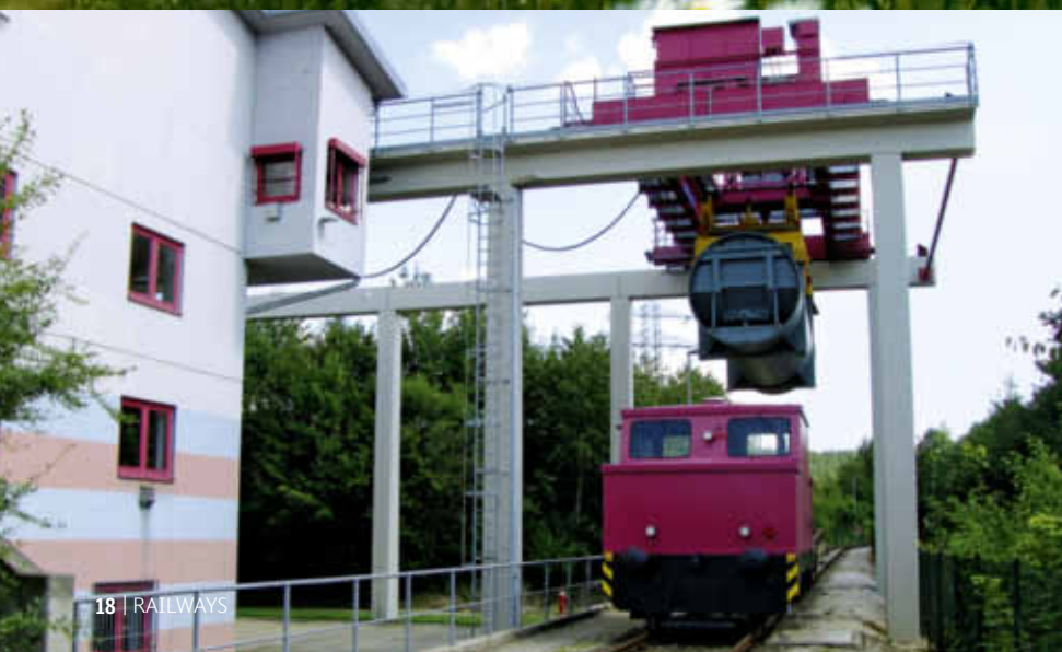
The Burgkirchen waste-to-energy plant incinerates over 220,000 tons of residual waste each year. Below: Unloading a special container at the waste-to-energy plant.
